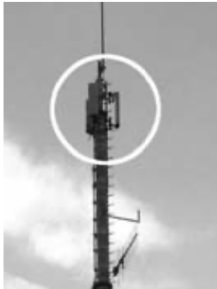
TETRA antenna (very similar to cell-phone antennas; three antennas are a characteristic feature).
