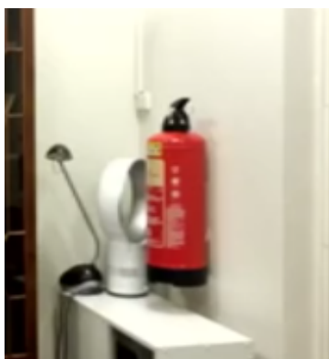
The fire extinguisher where a microphone was hidden
