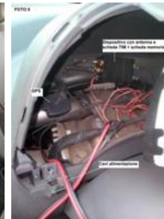
Counterclockwise from top: device with antenna, SIM and memory card; GPS; power cables
