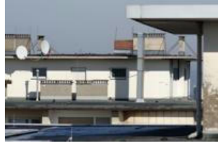
Power cable on the roof
